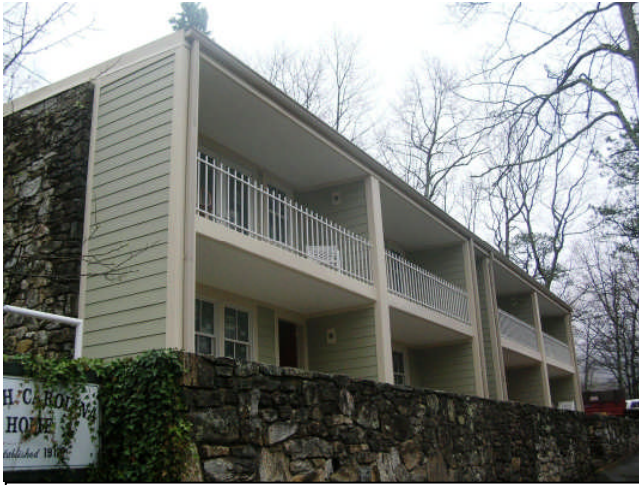
Front view of Kirk Apartments.
